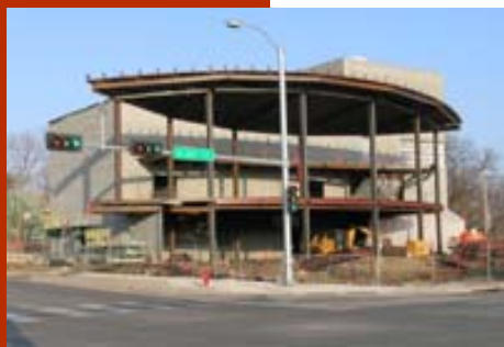
IQSC Building under construction
