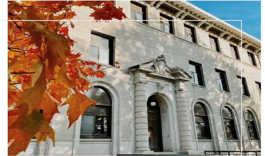
Filley Hall, East Campus
